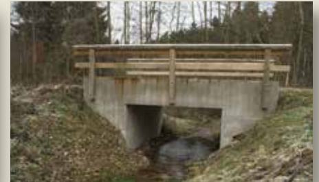
If access routes went over a stream, what was often used was sections of reinforced concrete.
