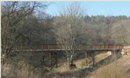
On Helingsbach stream, dam and canalisation pipes were removed and a wooden bridge put up for hikers, cyclists, riders and emergency vehicles.
