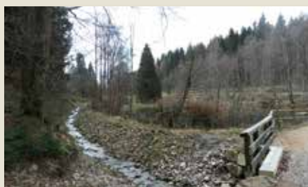
Where for wildlife conservation reasons it was desirable to retain ponds, the stream was led through a so-called 'bypass channel'.
