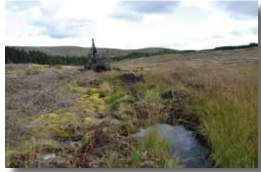
Above: Drain blocking in the Irfon Forest
